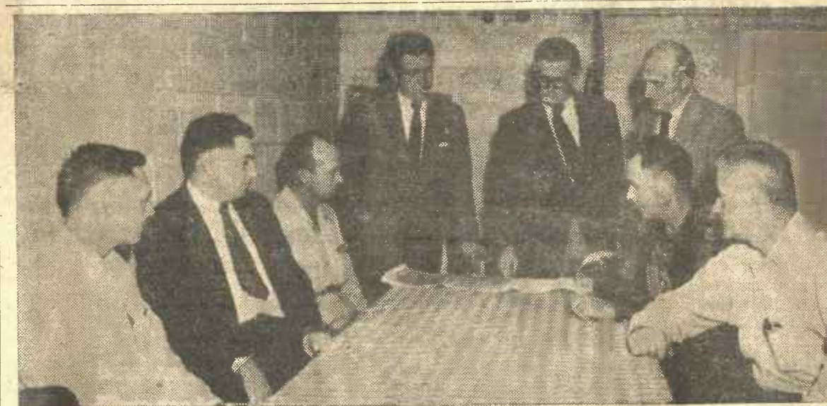
PLANNING HIGHWAY BEAUTIFICATION—This group of civic minded men are shown above as plans for beautification of the highways that pass through Iuka were discussed recently at the Country Club cafe. In the picture are, left to right, County Agent W. C. Hamilton, Reuben Grisham, Paul Edmondson, Bill Pyle, A. E. Holmes, Jr., of the State Highway Department, who outlined the department's methods of planting and caring for plants, Wayne Spinks, George Page, and Alver Belue. A sizeable amount of money has already been received to help pay for the plants and shrubs that the highway department has agreed to set out and help care for. (Staff photo)
